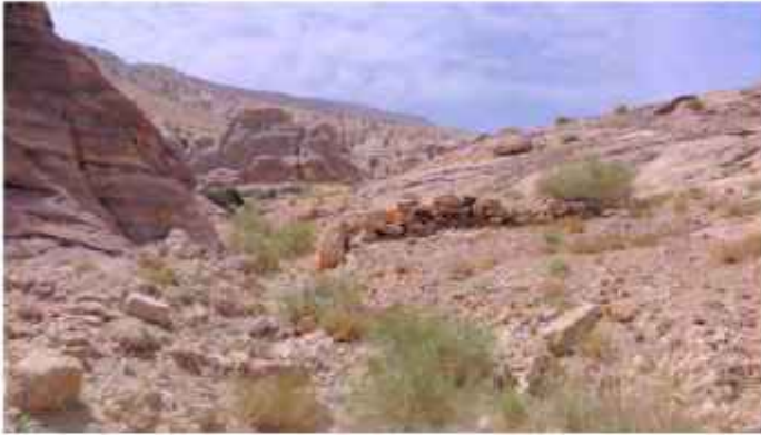
Dam 2 Before re-construction
