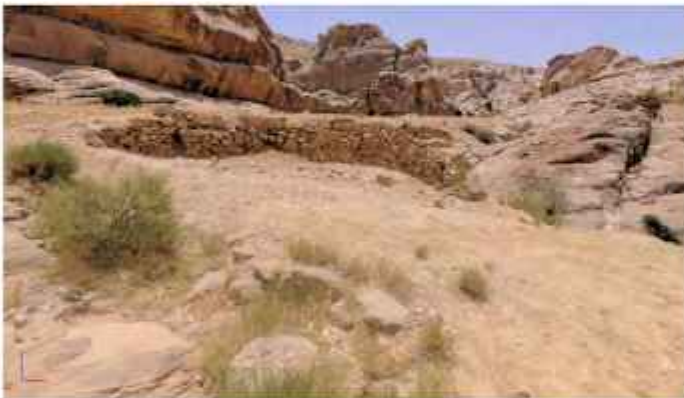
Dam 4 Before re-construction
