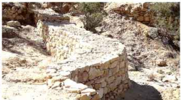
Dam 6 After re-construction
