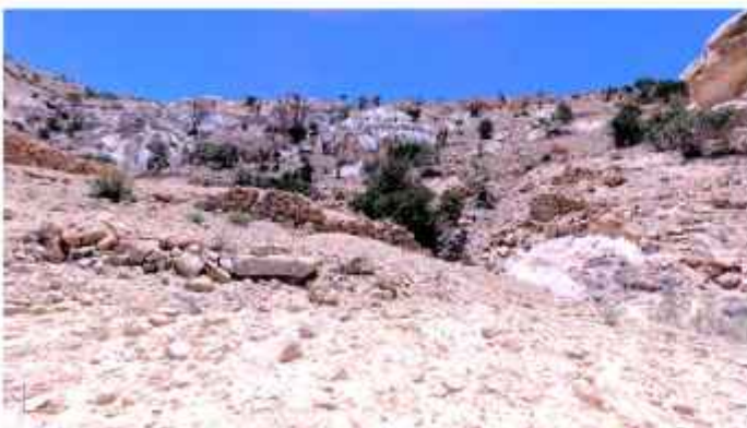
Dam 6 Before re-construction
