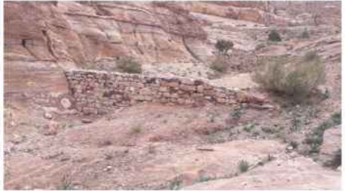
Dam 2 After re-construction
