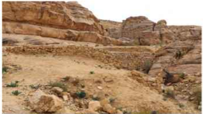
Dam 4 After re-construction
